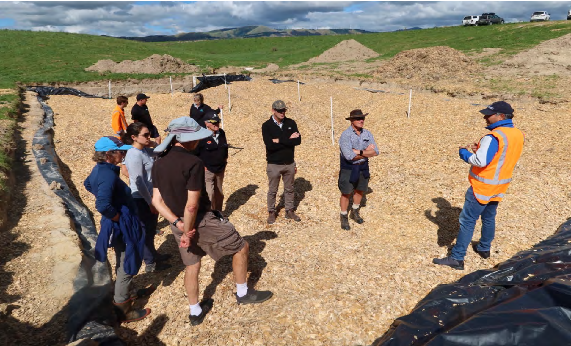
Construction of a woodchip bioreactor at Massey dairy No. 4
