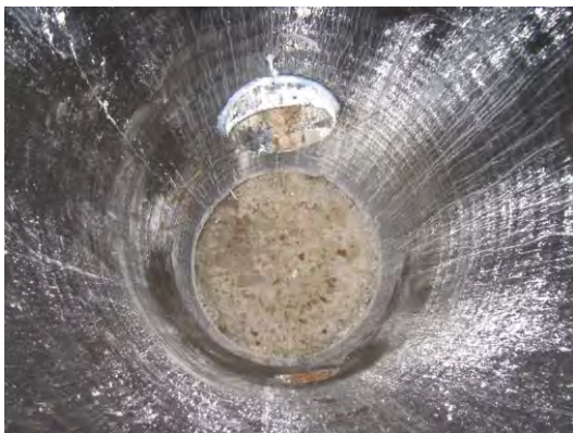
(c) Looking down the inside of the riser.
