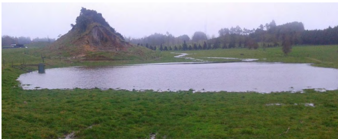
Figure 1 A Detainment Bund PS120 starting to fill during a run-off event. Lake Rotorua catchment.
