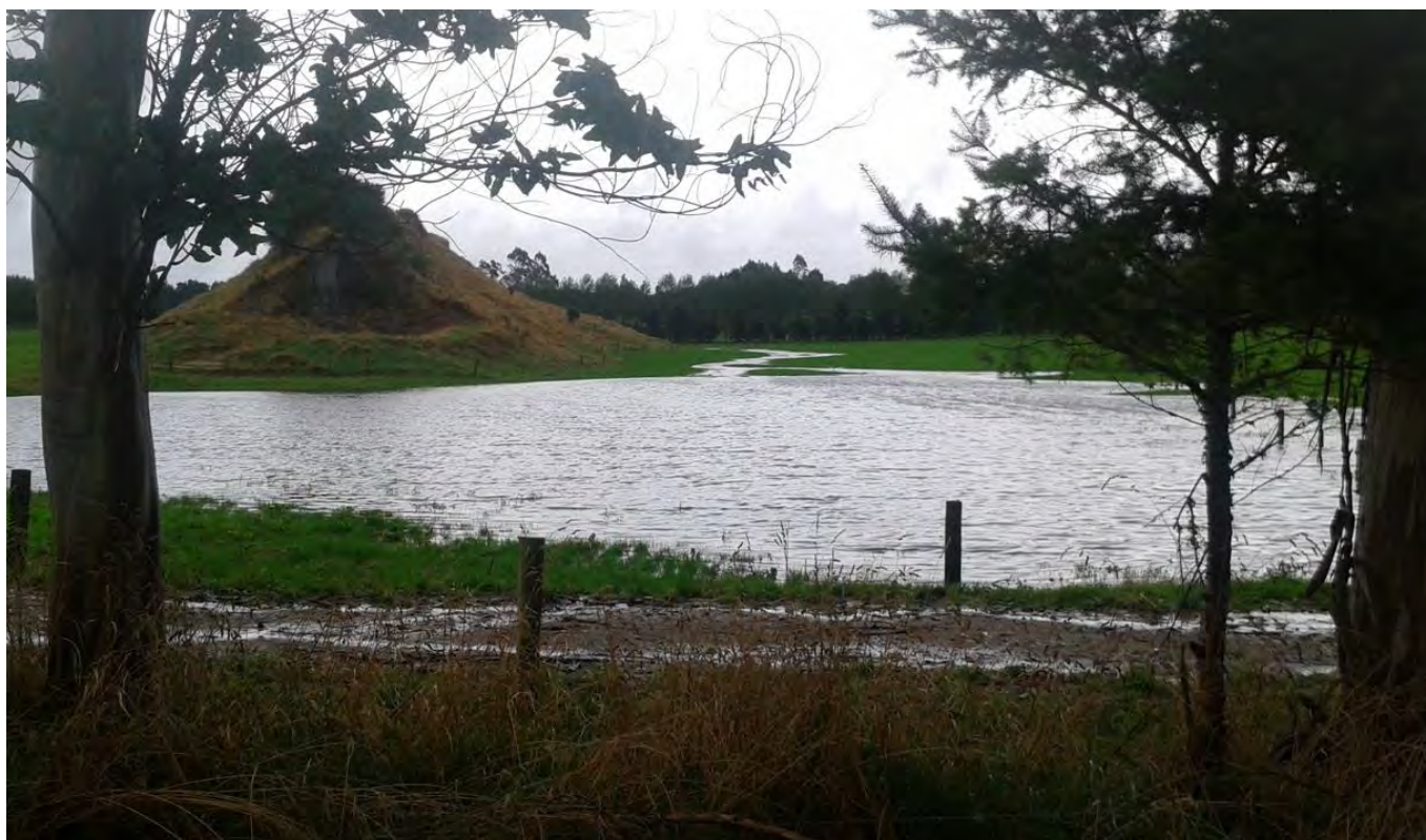
Figure 29 A storm water run-off event filling a Detainment Bund PS120 ponding area located on prime pasture. (Photo J. Paterson)
