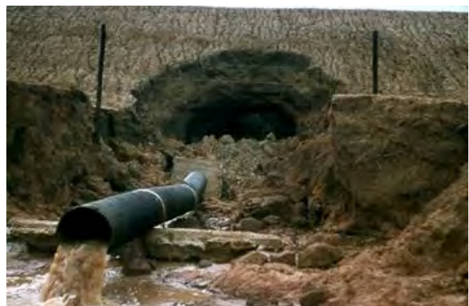
Figure 33 An example of ‘piping’ erosion. Poor pipe haunching, inadequate compaction around the pipe during installation, causing embankment failure. (Pipe cross section diagram and photo from FEMA 2005).
