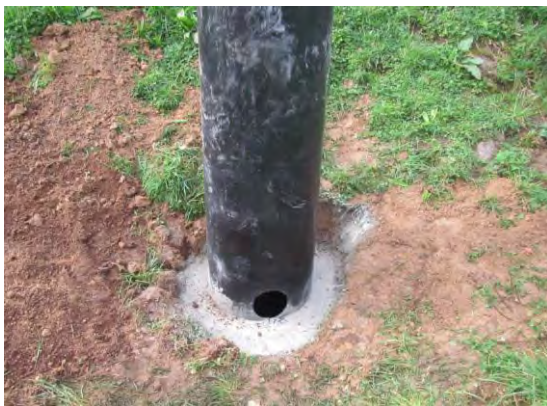
(a) Front view of a fitted upstand riser.
