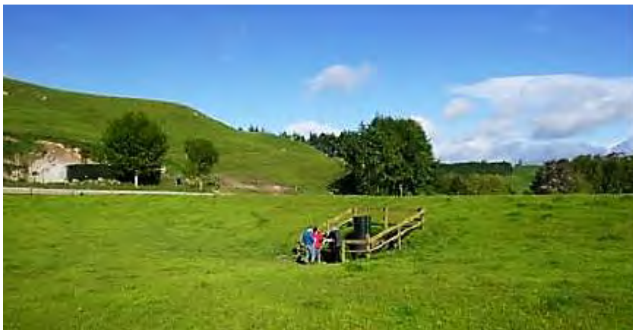
Figure 35 A typical Detainment Bund PS120 on prime valley floor pasture.
