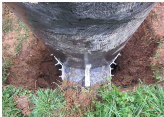
(b) Rear view – pipe/riser joint.
