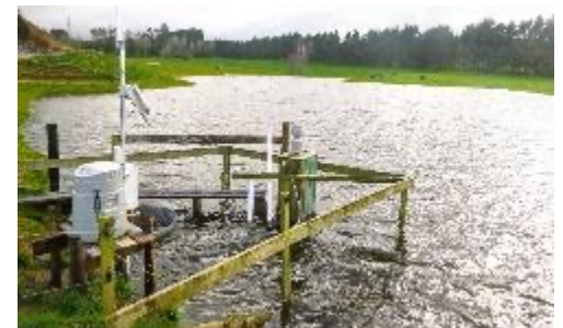
Sediment detention bunds
