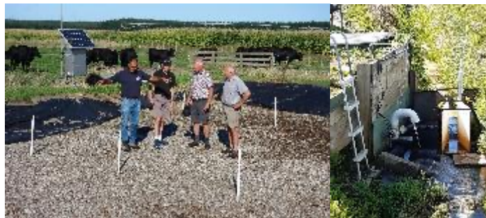
Woodchip bioreactor treats drainage waters
